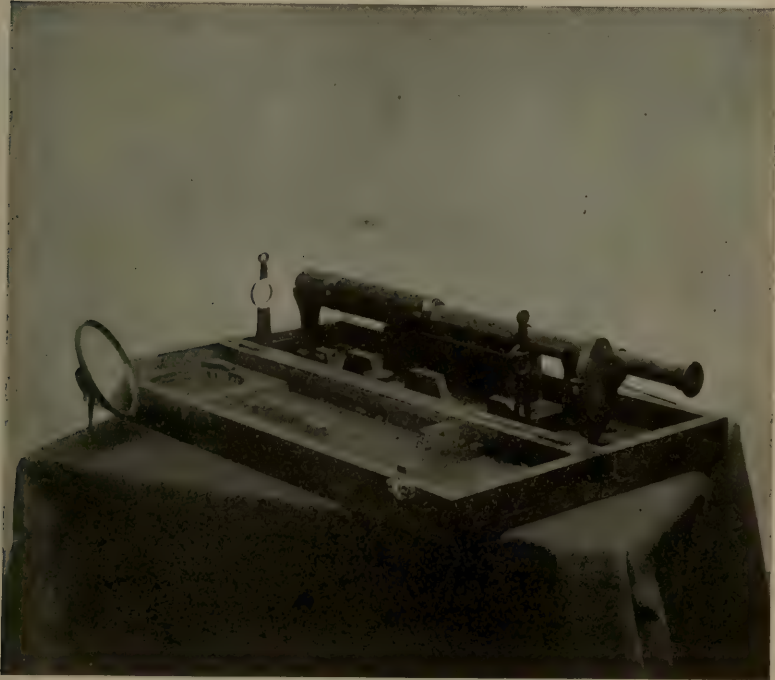
FIG. 14. Box Heliotrope. (Coast and Geodetic Survey.)
